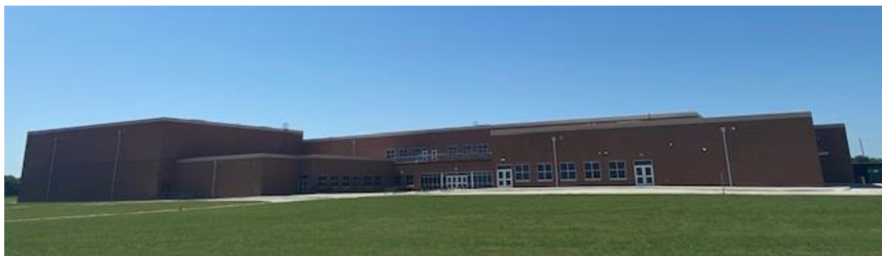
Figure #8. Back of the newly built Tioga High School. April 10 th , 2020.
