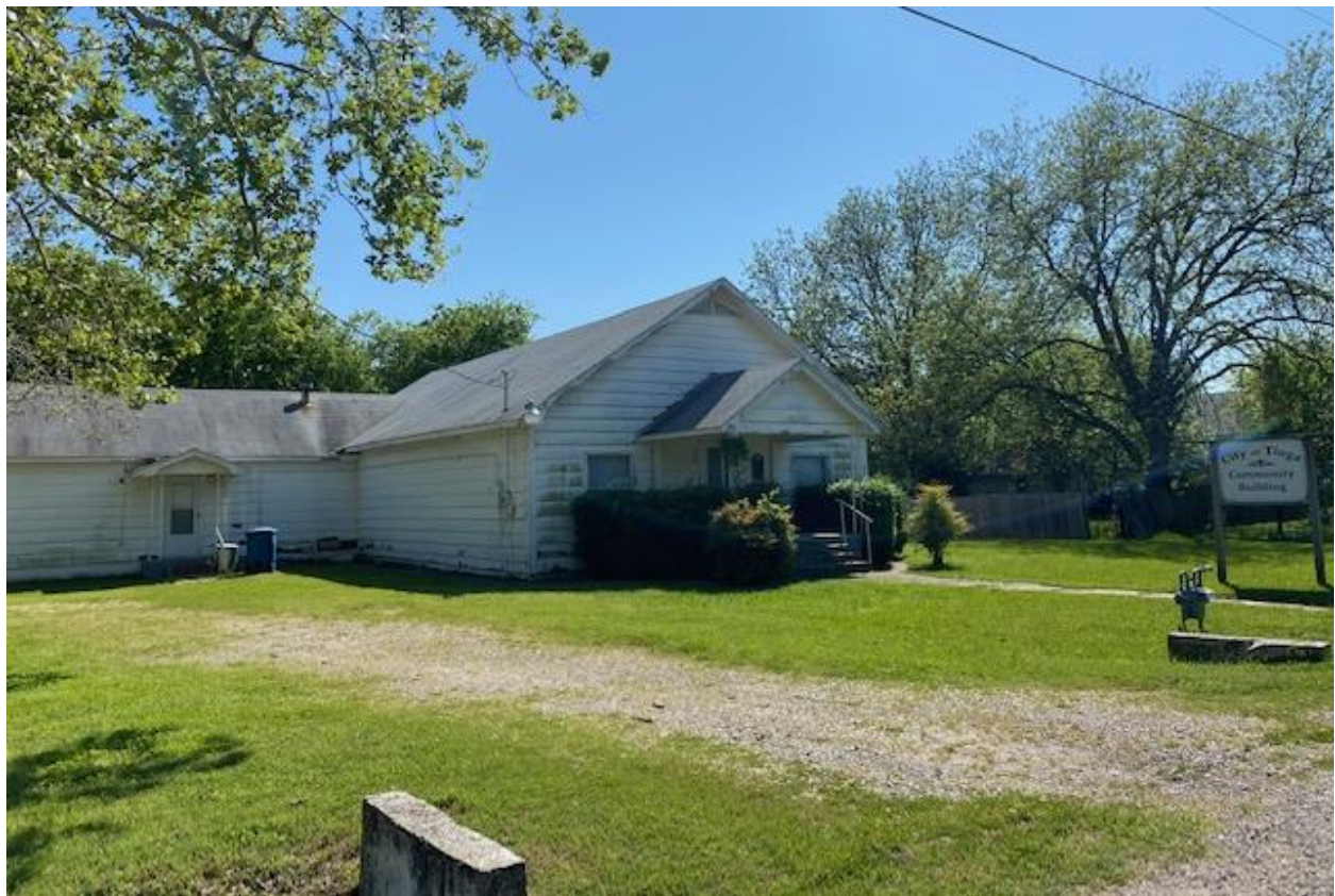
Figure #1. Community building established in an older building without renovations. April 10 th , 2020.
