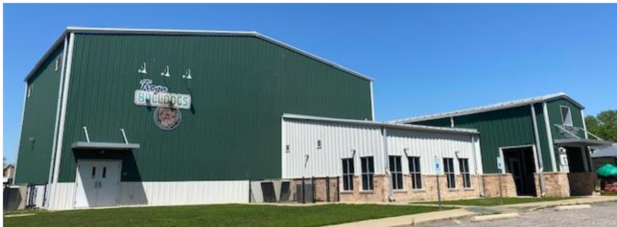
Figure #13. Tioga Child Development Center (Pre-K) attached to Tioga Elementary and Middle School campus. April 10 th , 2020.
