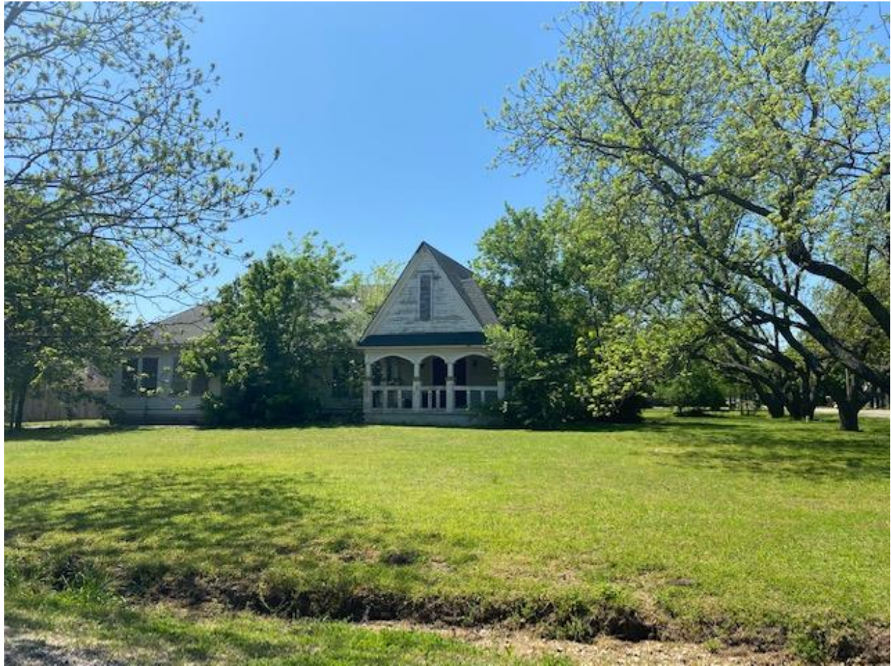
Figure #6. Example of one of the sparsely located dilapidated homes. April 10 th , 2020.
