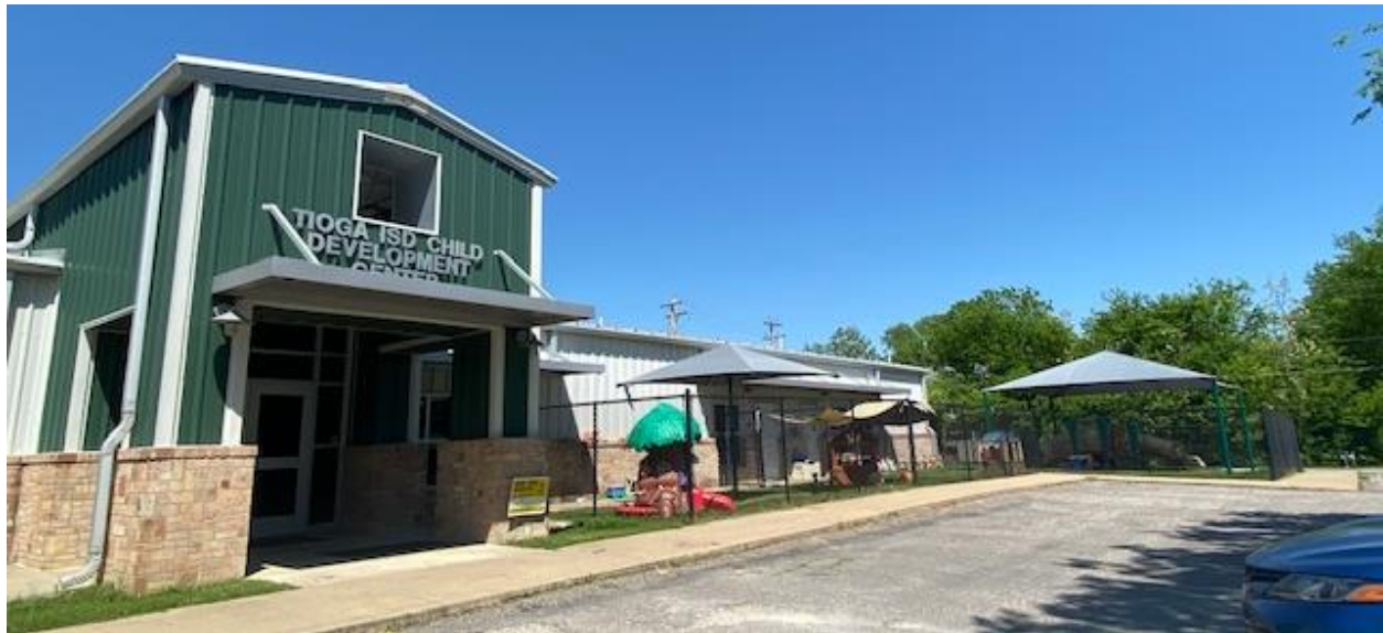
Figure #12. Close up of Tioga Child Development Center (Pre-K) attached to Tioga Elementary and Middle School campus. April 10 th , 2020.
